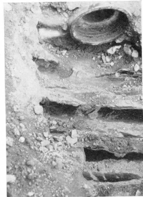
DAMAGE TO DUCT ROUTE CONTAINING HIGH WYCOMBE-LONDON No. 2 CABLE
