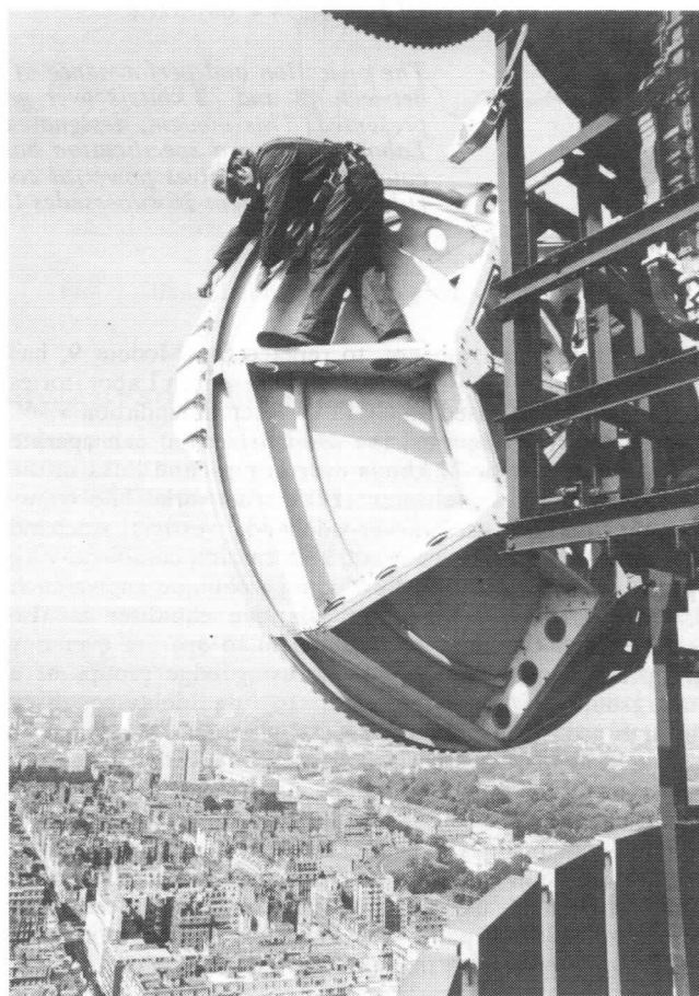
FIG. 2—Adjustments being made to one of the new dish aerials mounted on the London Telecom Tower
